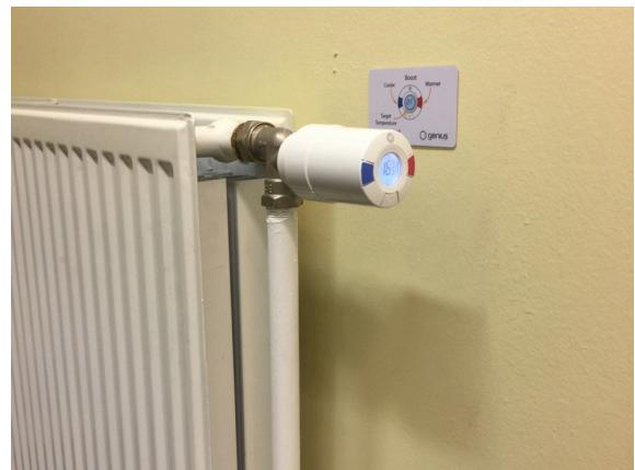
Genius Radiator Valves, replaced existing TRVs
