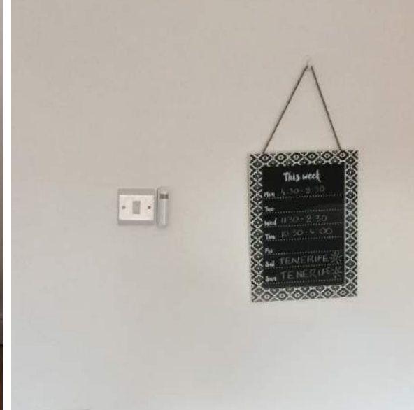
From left to right: Bernard Sampson pointing to a Heat Genius valve. The whole system is wireless, making it unobtrusive and quick to install. | The small sensor near the light switch allows Heat Genius to detect when this bedroom is empty, and turn off the radiator automatically. | Even shared areas of the house, which often have complex usage patterns, can be controlled automatically.
